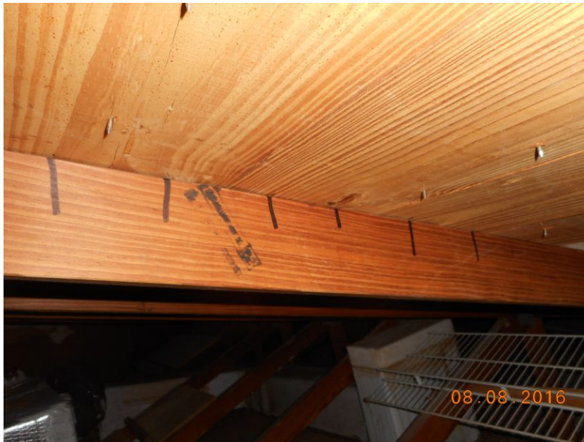
Dimensional Lumber/Tongue & Groove Decking with 2 nails per board
