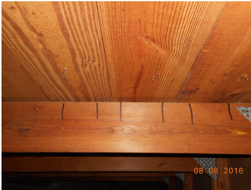
Dimensional Lumber/Tongue & Groove-2 nails per board
