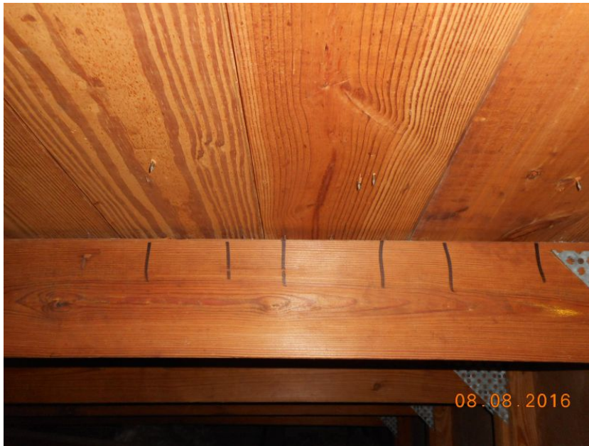
Dimensional Lumber/Tongue & Groove-2 nails per board
